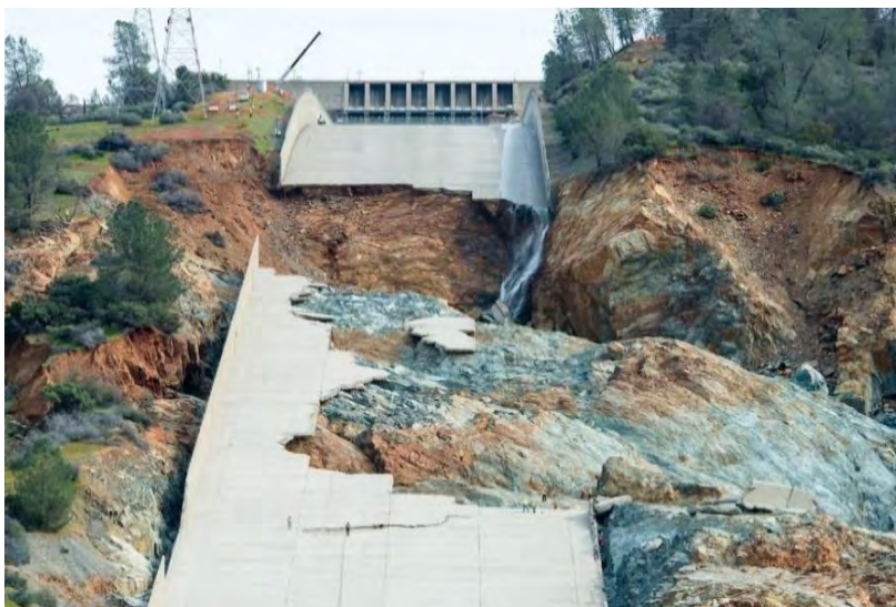
Figure 4-23. Oroville Dam Spillway after 2017 failure.
