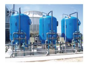
Series installation allows media to be replaced without shutting down the well, which is beneficial to the water distribution system, especially during peak demand periods.
